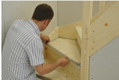
Almost any required shape can be created due to the different aluminium rails
