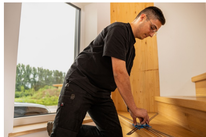
Simple scanning of the shape of steps.
