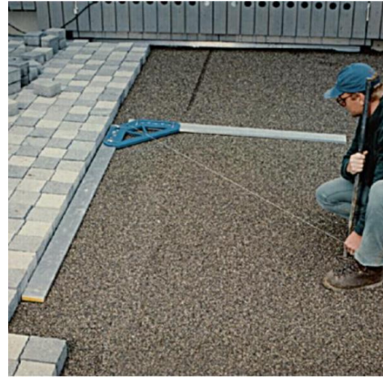
Connects two straightedges to form a right angle
