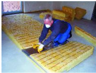
The insulation gauge is adjustable in width and length and can be loaded with body weight when cutting to size.
