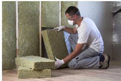
Fast and accurate cutting of insulation materials
