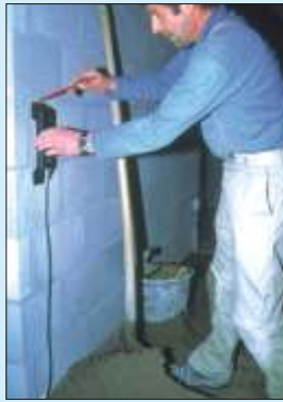
Transfer the zero level around the corner
