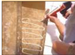
To fix the step you just put the special glue in snake line on the old and the new step.
