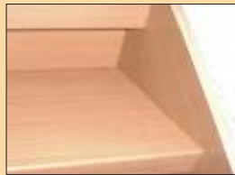
A thin silicon line is enough to make the rabbet invisible; and the stair comes out like new.
