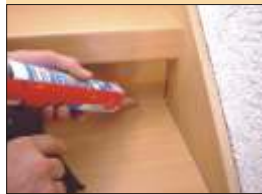
After the step and the stair riser are fixed you have to close the rabbet with coloured silicon.
