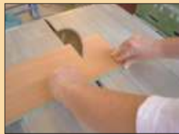
Step-by-step: The end of the stair rise will be cut in a 45° angle.
