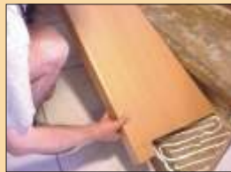
The new step has to be put down and pushed back with the fist or a special hammer.
