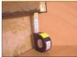
After this you have to mess the altitude, the length, and the angel on the right and left side of the stair riser.
